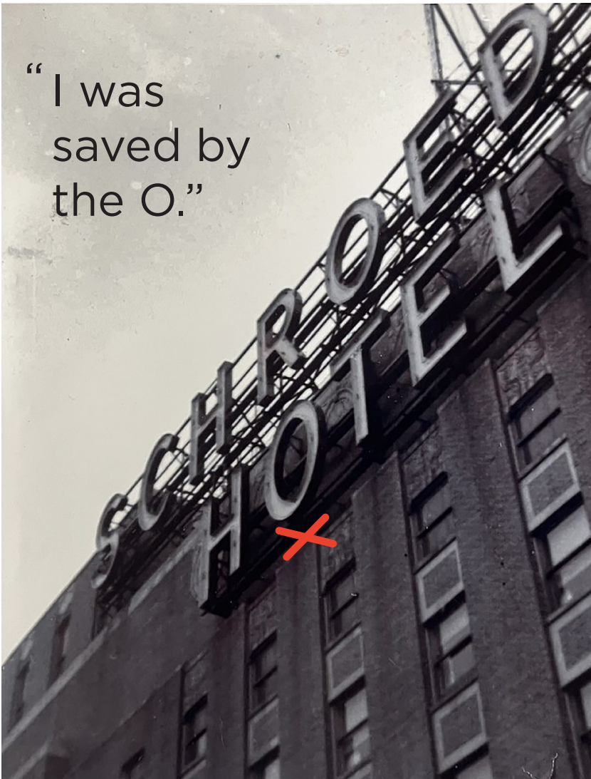
The red X marks the spot where Dean was hanging in a rain storm on a 27-story building.
